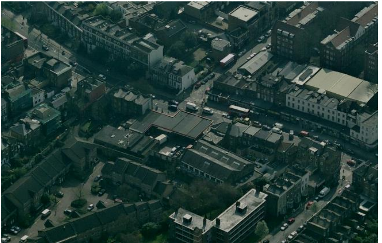
Photo 4: Aerial view from East
