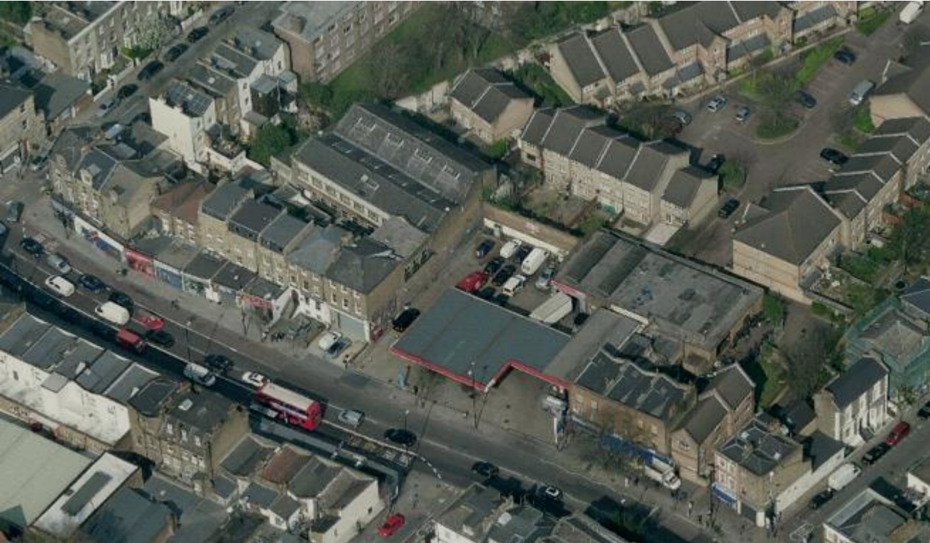
Photo 1: Aerial view from West
